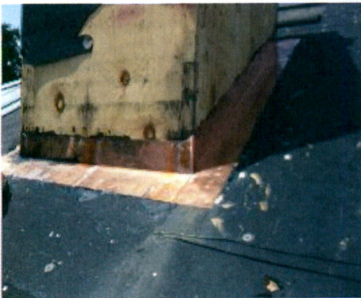
Flashed the entire perimeter of structure.
