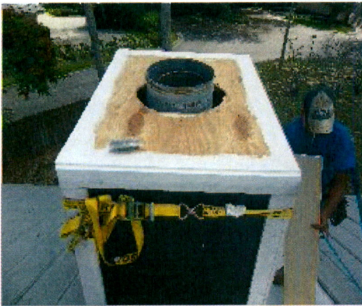
Solid plywood on top, sealed perimeter to avoid potential blow in during high wind driven rains.
