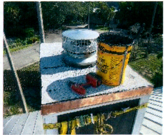
Roof on top in lieu of cap, will not blow off as caps do. New spark arrester provided.
