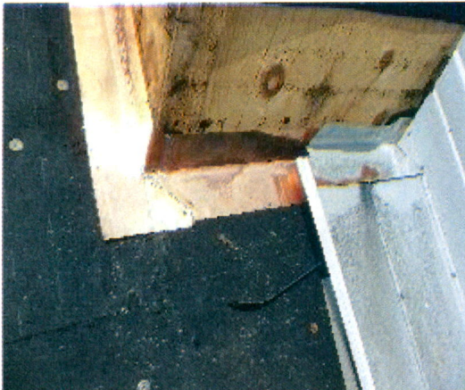
Typical flashing, all corners soldered, then the top of the flashing sealed direct to sheeting
