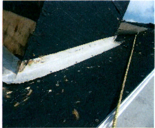
Original flashing installation over the felt
