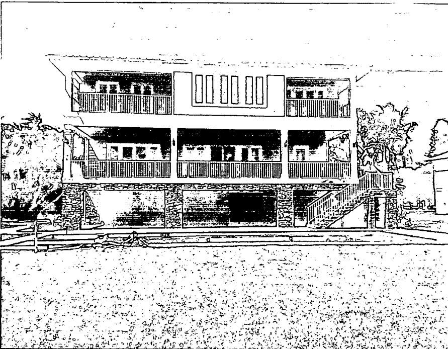
REAR VIEW - PHOTO TAKEN MARCH 28, 2015
